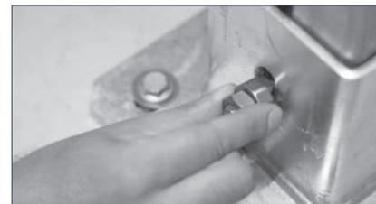
Insert T-lock plus through component and profile, position as required.
